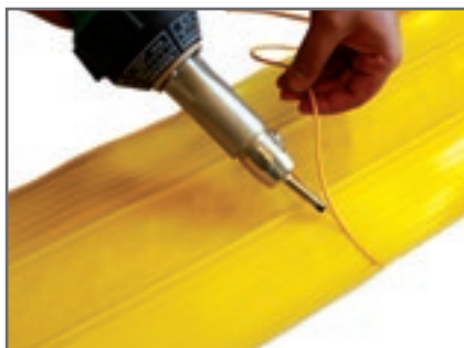
Hot air blower welding procedure
