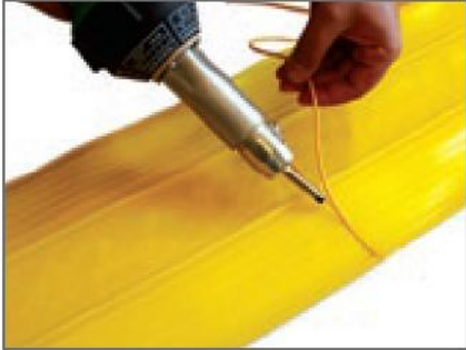
Hot air blower welding procedure
